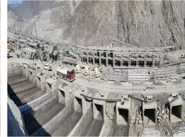
Diamer Basha Dam
